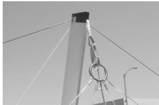
Check the condition of the sweep wires in the vicinity of the kingpost base bracket.
